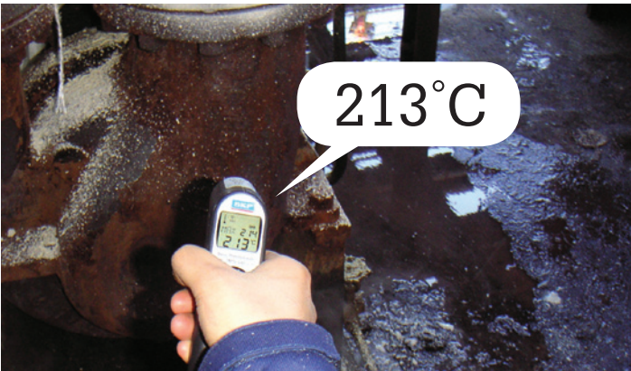
Temperature on the pipe before HPC® Coating was 415.4°F
