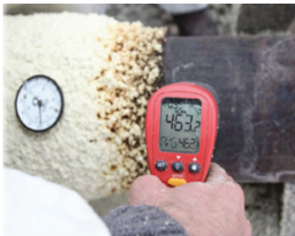
Before HPC® Coating application 865.4°F (463°C)
