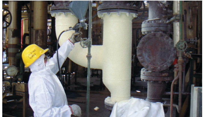
Phase of HPC® Coating application
