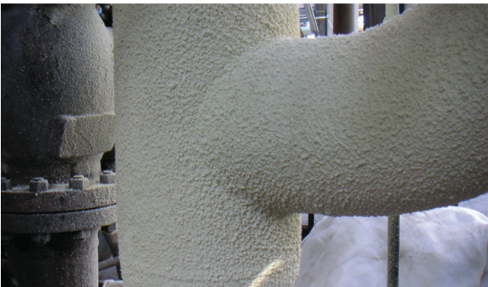
Finished HPC® Coating application
