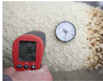
After HPC® Coating application 96.8°F (36°C)
