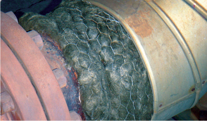
Exposed traditional wrap and cladding insulation
