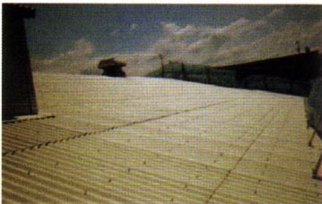
Application of REINFORCE BASE
